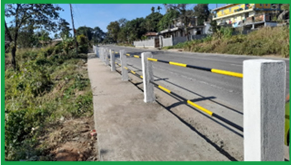
Construction of footpath beside NH 6 in Thangskai village
