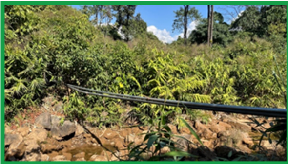
Replacement of damaged drinking water pipeline to Lumshnong village
