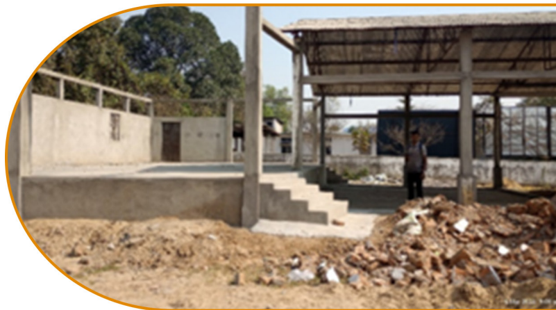
Construction of Community Hall
