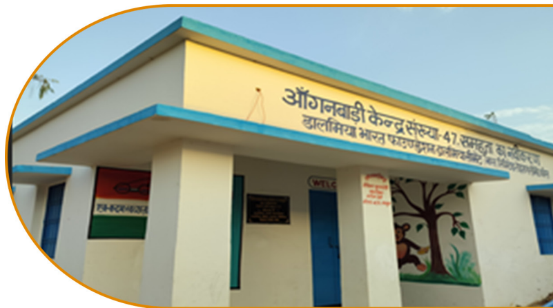
→ Anganwadi renovation at Samahuta village
