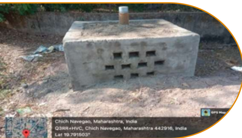
Borewell Recharge Pit
