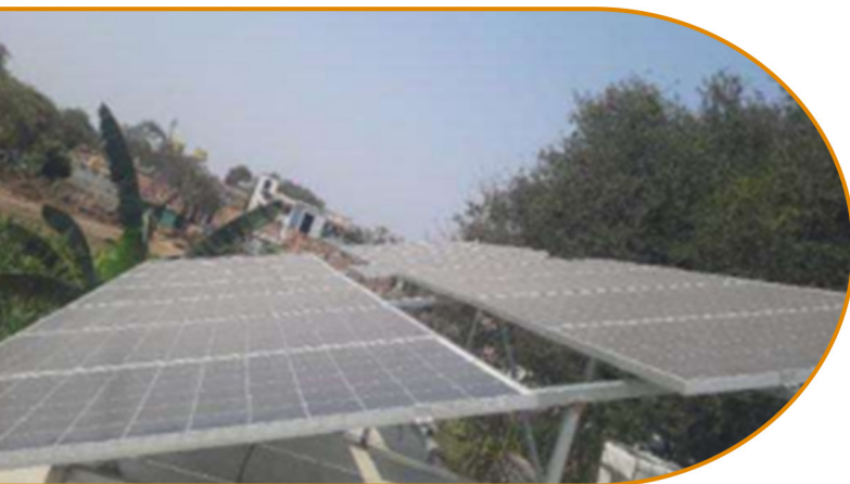
→ Solar Unit Installation of 5 KW of capacity
