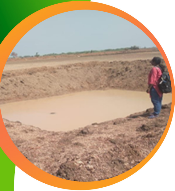
Farm pond constructed under Manami Watershed Project
