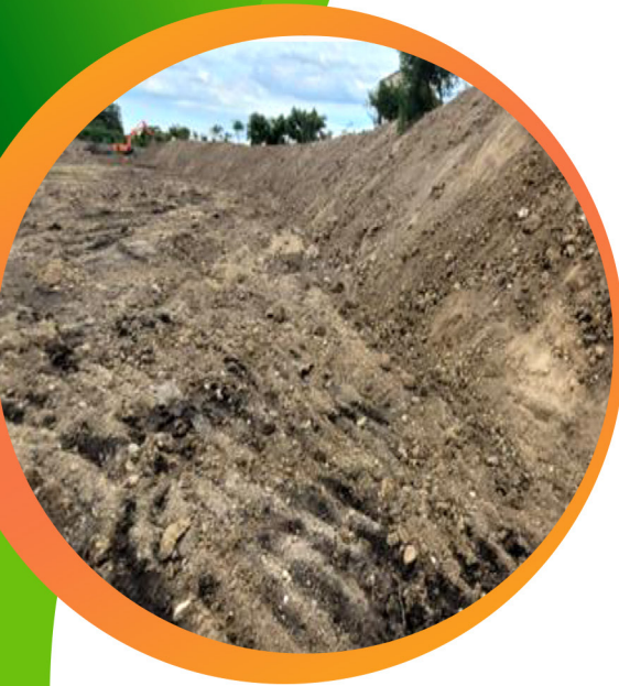
Village pond desilted and bunds strengthened at Thamaraikulam
