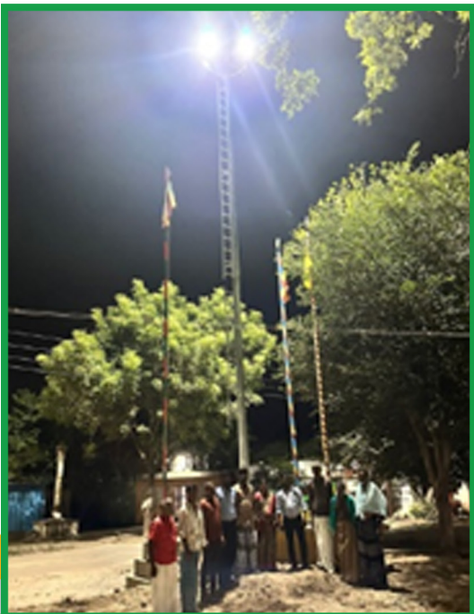
Installation of tower lights
