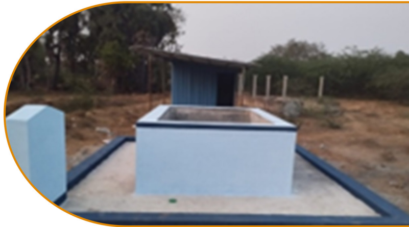
Water tank construction for Periathirukkonam Panchayat
