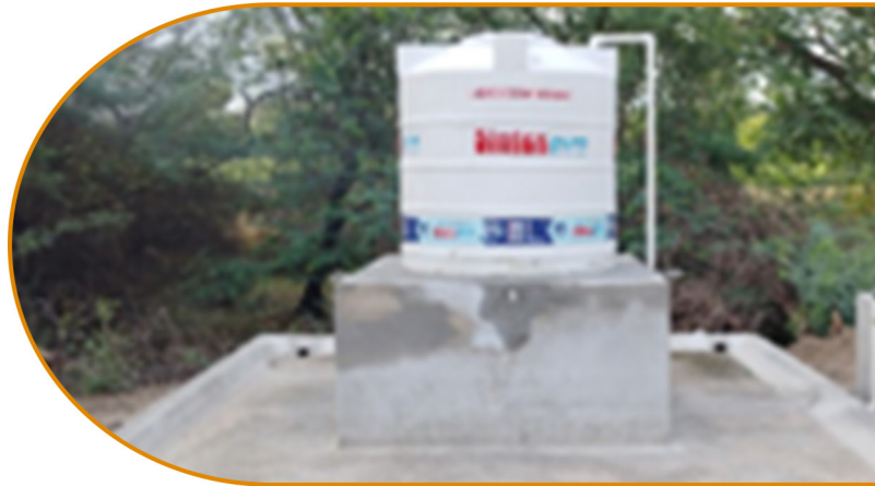
Multipurpose water tank construction for Kayarlabath Panchayat
